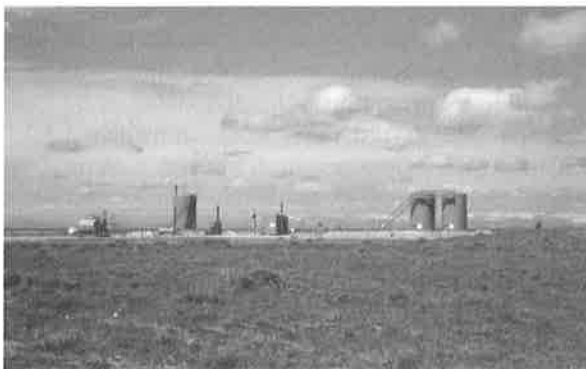
Gas wells on the Pinedale Mesa.
